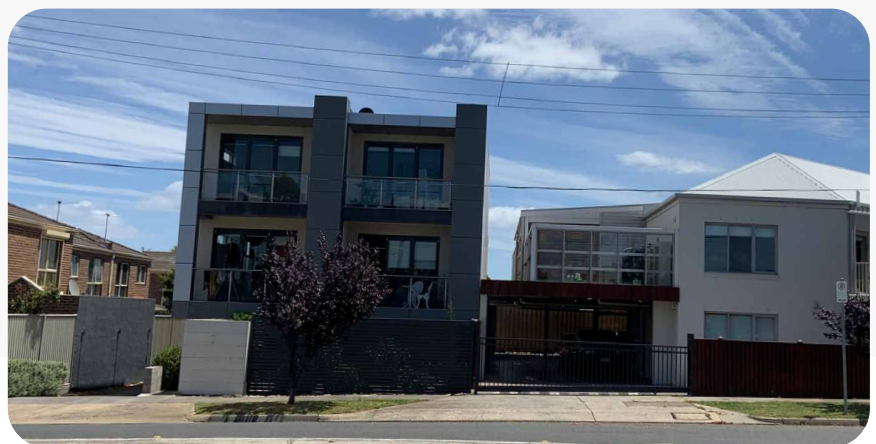
Recent multi-dwelling building, providing little streetscape amenity, activation or interest.
