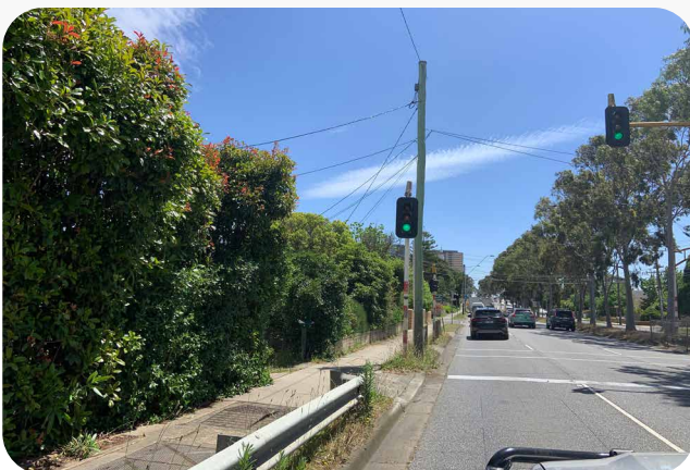
Lack of pedestrian amenity along sections of Springvale Road where no service road is provided
