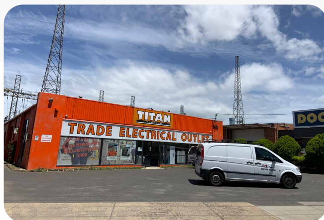
Large front setback, with no tree planting or landscape amenity to the street - limited edge planting around the car park.
